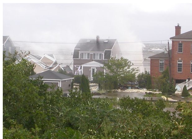
FIGURE 4. Cosey Beach during Hurricane Irene. Note collapsing house on left and wave splash overtopping house in center. (Photo courtesy of James Tait.)
